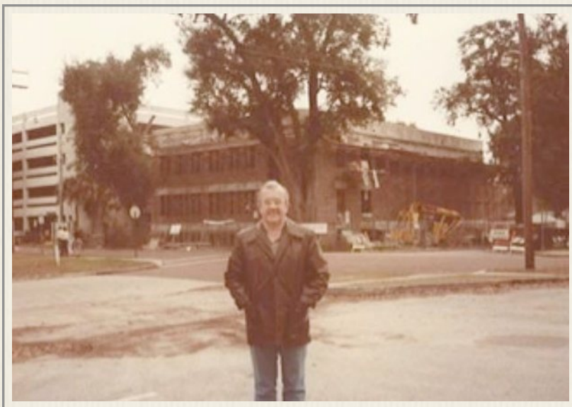
Tom in front of Medical Examiner Office under construction, 1984
