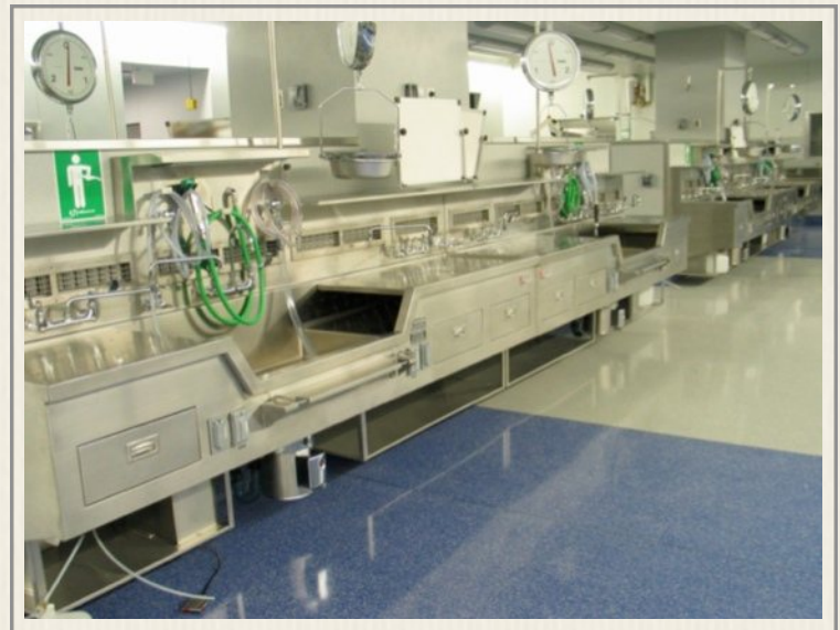
New autopsy room
