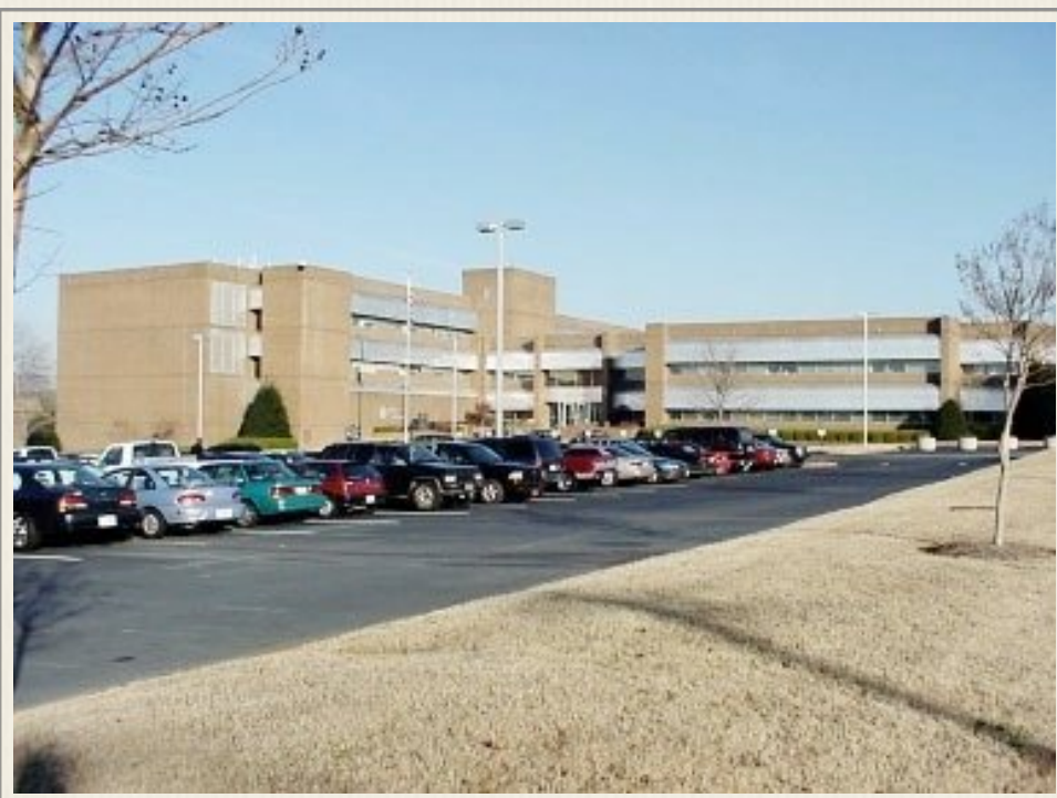
GBI and DOFS Headquarters constructed in 1984. Panthers- ville Road, Decatur.
