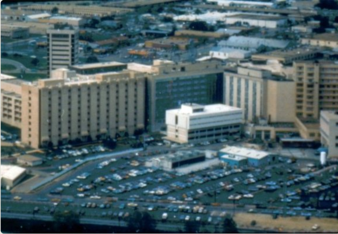
Aerial view of SWIFS with top two floors added
