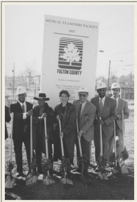
1997 Ground breaking for the new FCME facility to be built at 430 Pryor Street SW, Atlanta. Saleh Zaki (third from right) wields a shovel at the ceremony.
