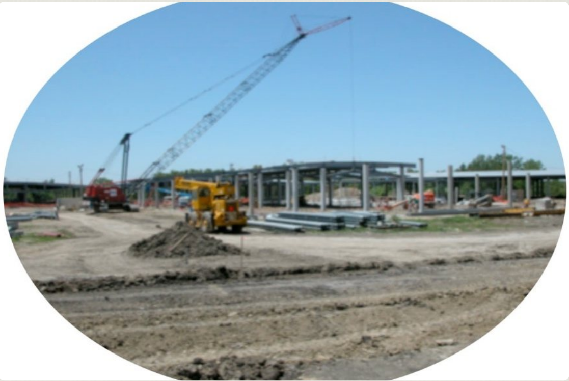
Construction of the facility
