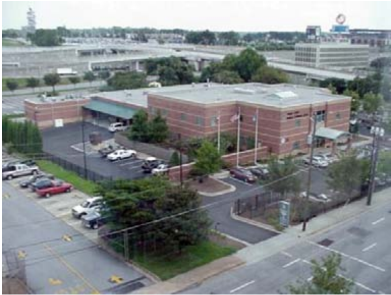
33,000 square feet, 3-building Fulton County Medical Examiner's Center which opened in April of 1999. Randy Hanzlick has been the only Chief ME to serve in this facility.
