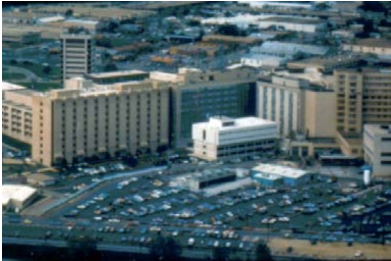
Aerial view of SWIFS with top two floors added
