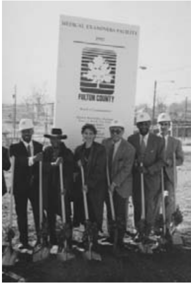
1997 Ground breaking for the new FCME facility to be built at 430 Pryor Street SW, Atlanta. Saleh Zaki (third from right) wields a shovel at the ceremony.
